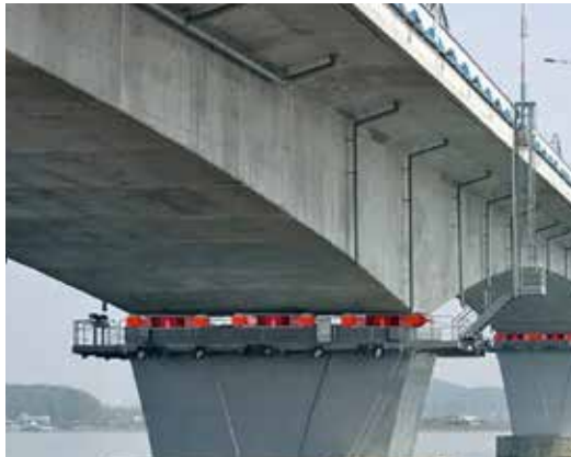
Bridge Bearing & Expansion Joints
